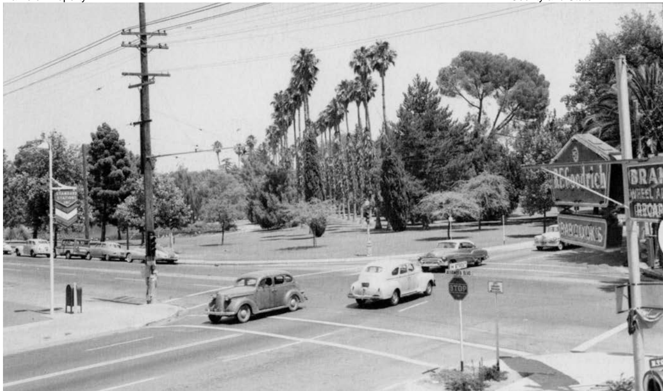
Figure 22. Circa 1953. Intersection of Alhambra Boulevard and H Street. Palm Drive roadway has been removed and replaced with lawn, but the allée of palms is still very prominent. The additional parking and roadway at this corner of the park is yet to be constructed. Center for Sacramento History.
